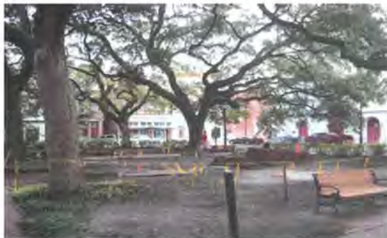
Repairs in Wright Square
