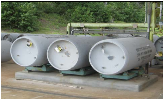
Chlorine gas tanks at the I & D Plant
