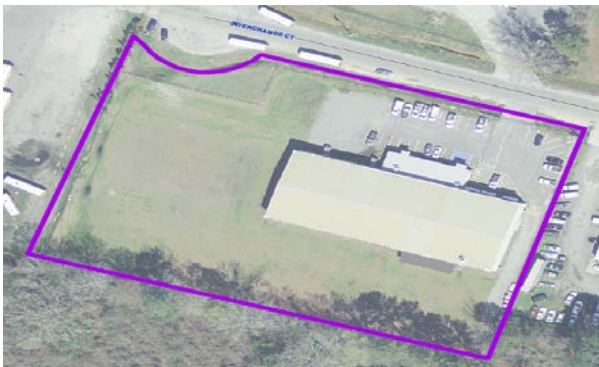
Park and Tree Maintenance Building
