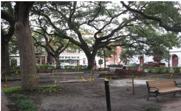
Repairs in Wright Square
