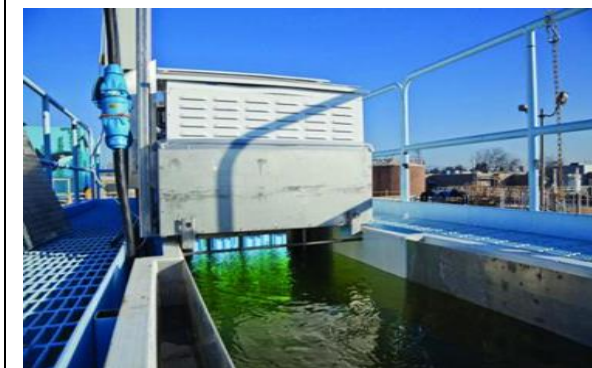
Discharged water passing through a UV disinfection station
