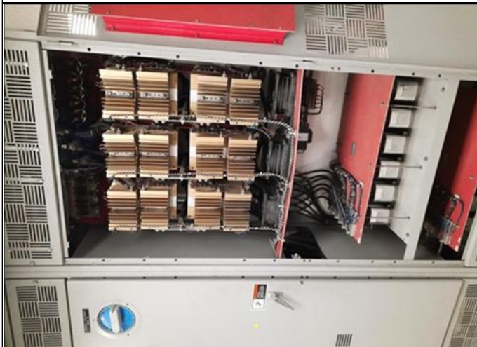
Variable Frequency Drive Cabinet
