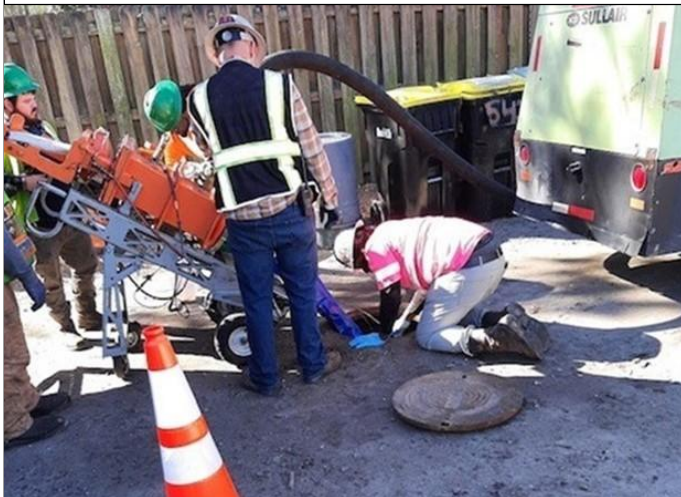
Sewer Line Rehabilitation
