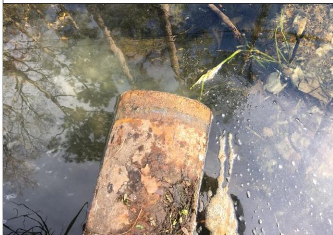
Wilshire Canal to Vernon River Sewer Main
