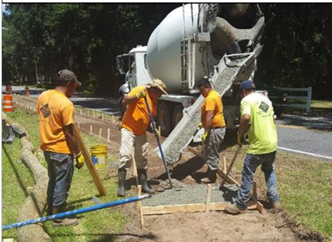
New Sidewalk Installation
