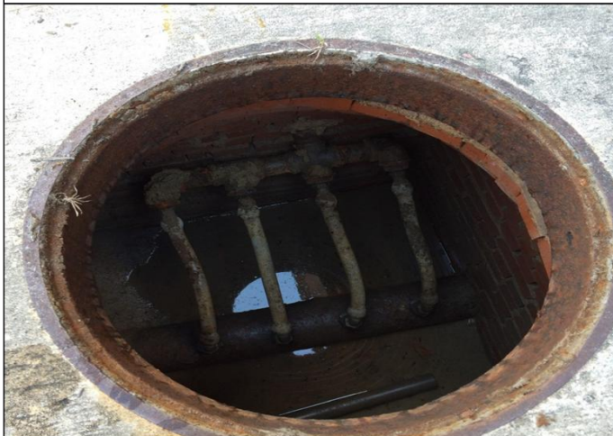
Water Service Gooseneck Connections to Main
