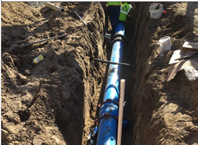
Typical Water Main Replacement
