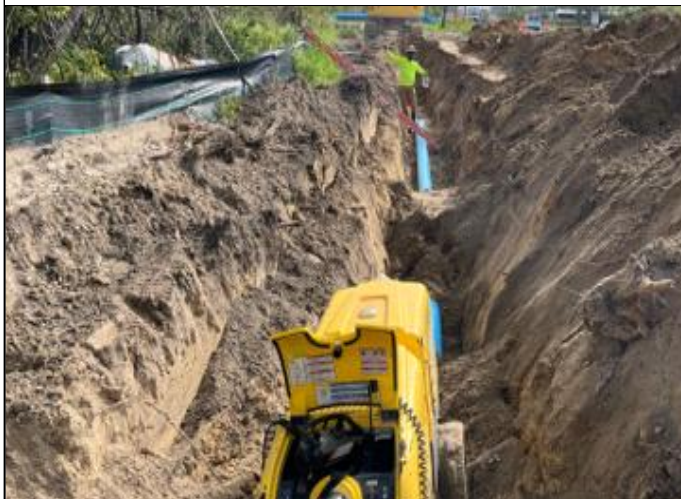
Compacting Backfill over Pipe Joints
