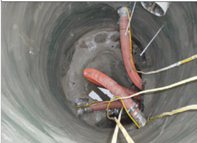
Lift Station Rehabilitation
