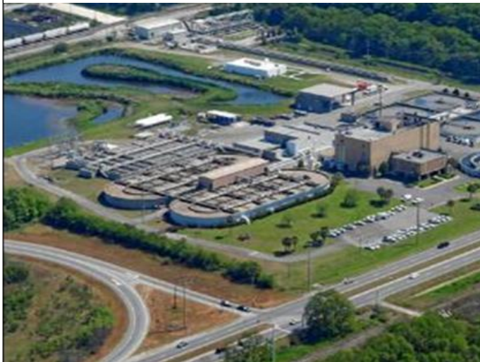
President Street Water Reclamation Facility
