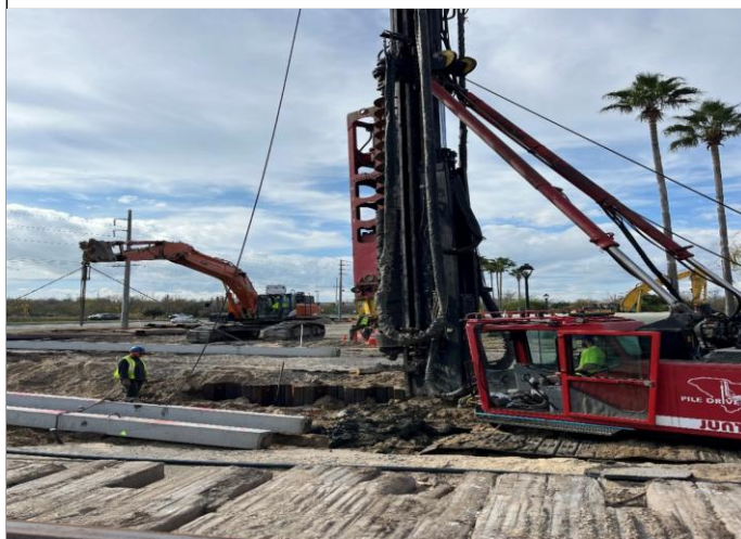
Gravity Thickener Re-build
