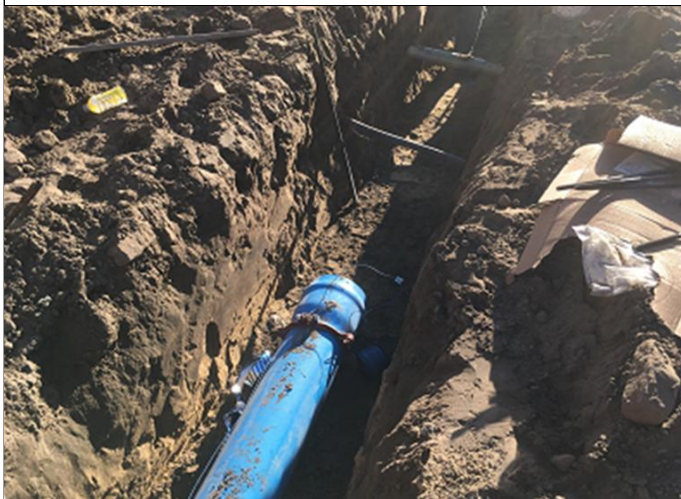
Water Main Repair
