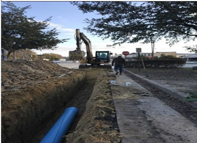
12" Water Main Installation
