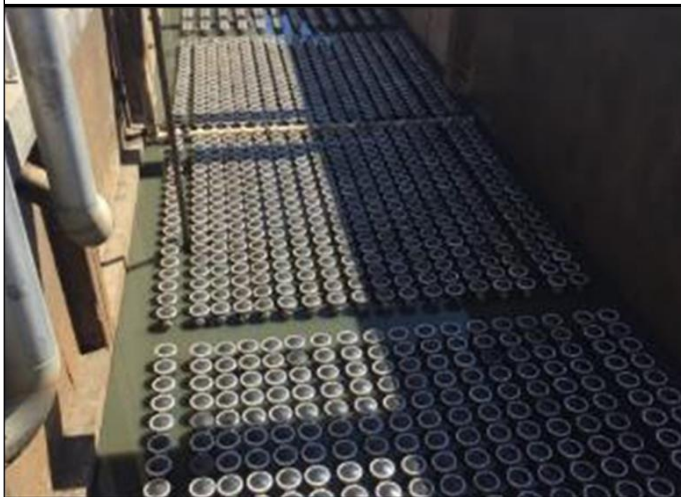
Zone 3 of 6 Diffusers in #1 Aeration Basin
